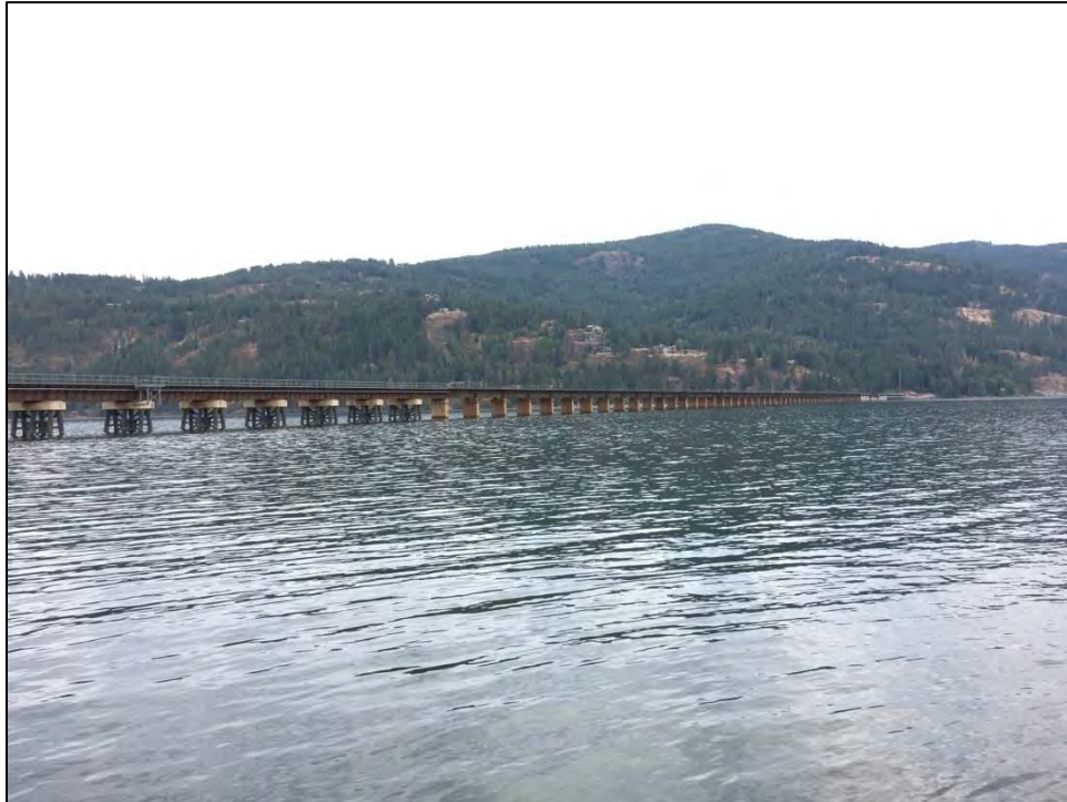
Figure 30. BNSF Bridge 3.9, West Elevation
