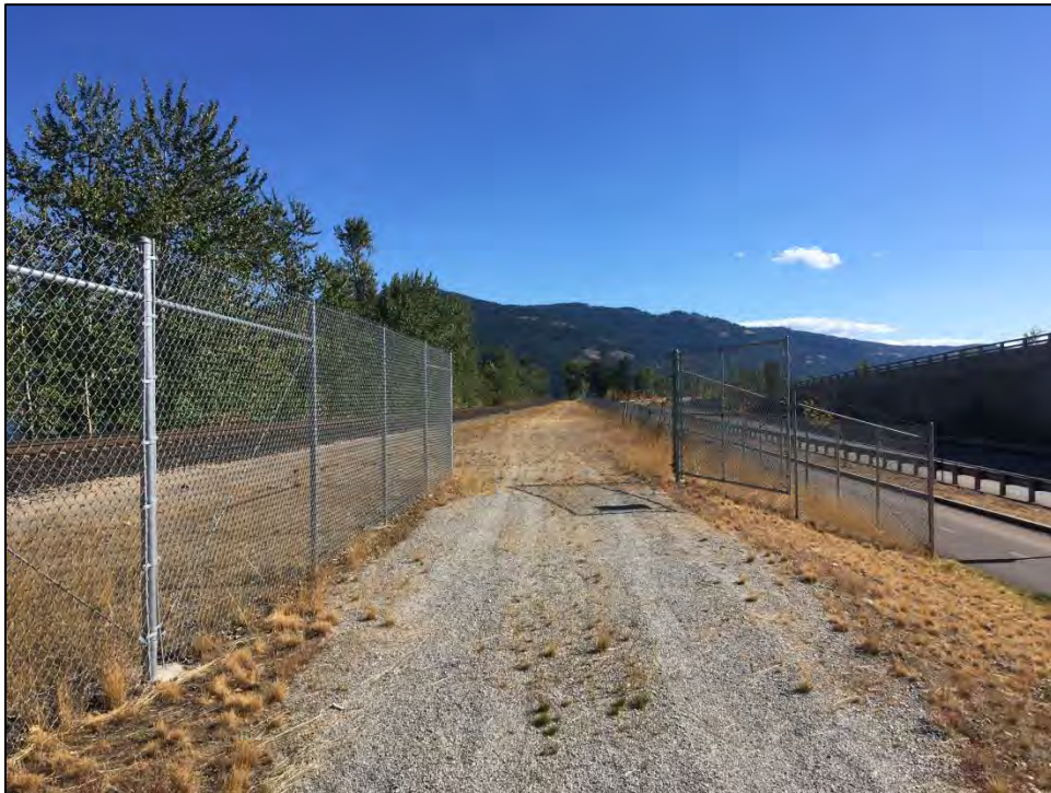
Figure 12. New Fill Prism East of US95, South of Bridge 3.1; View to South
