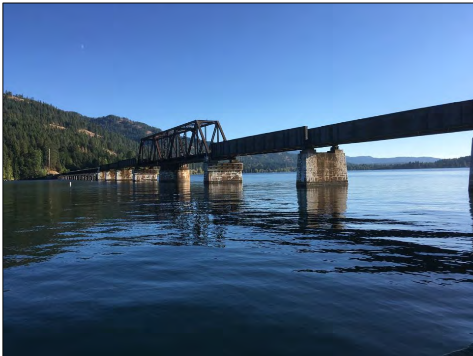
Figure 31. BNSF Bridge 3.9, East Elevation, South Half
