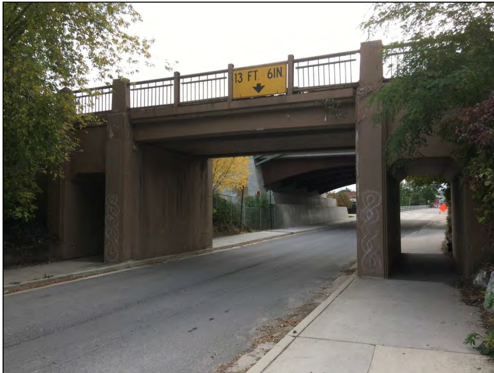
Figure 28. BNSF Bridge 3.0 West Elevation
