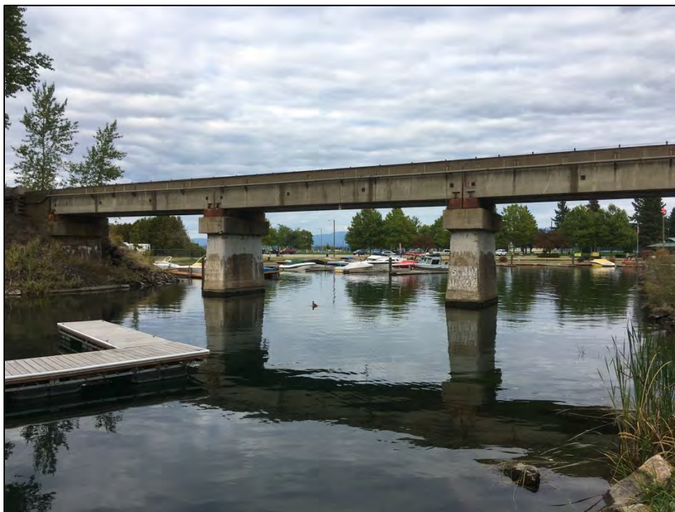
Figure 32. BNSF Bridge 3.1, West Elevation
