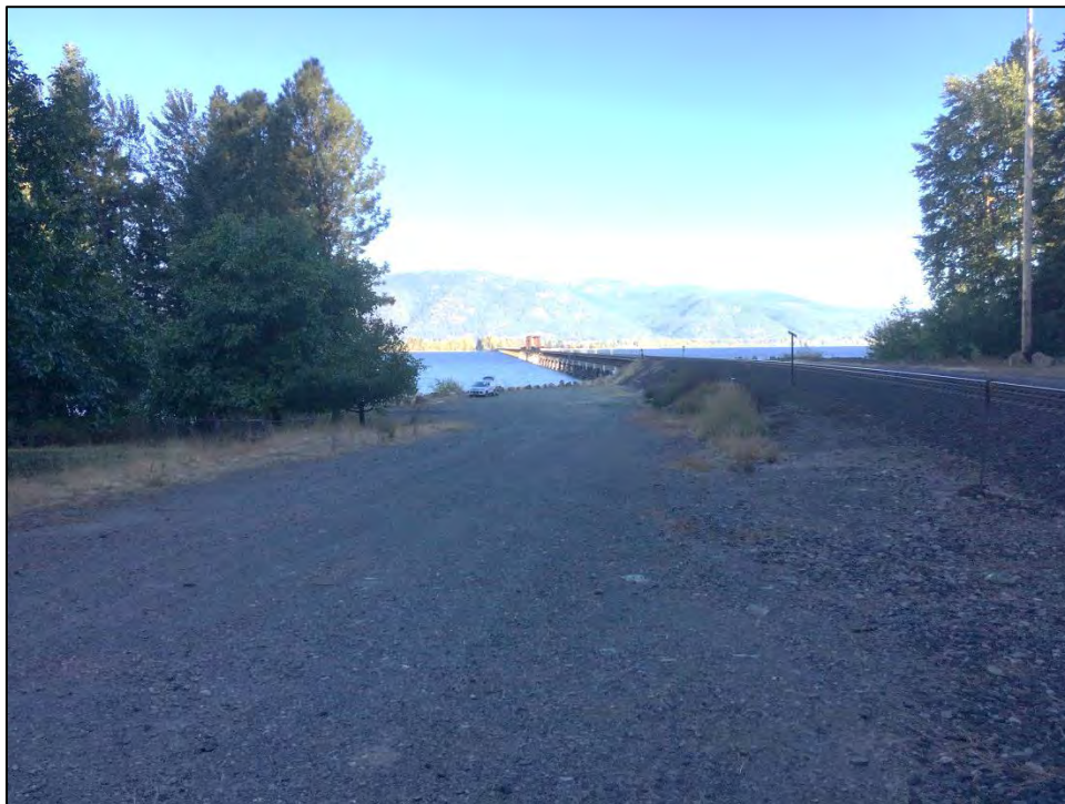
Figure 2. View of conditions south of 10BR38, showing modifications since 2008; view northeast.
