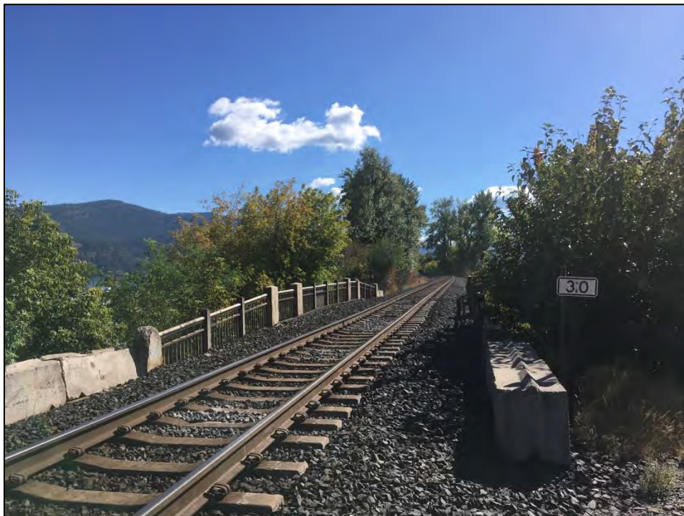
Figure 29. BNSF Bridge 3.1 Railing; View South
