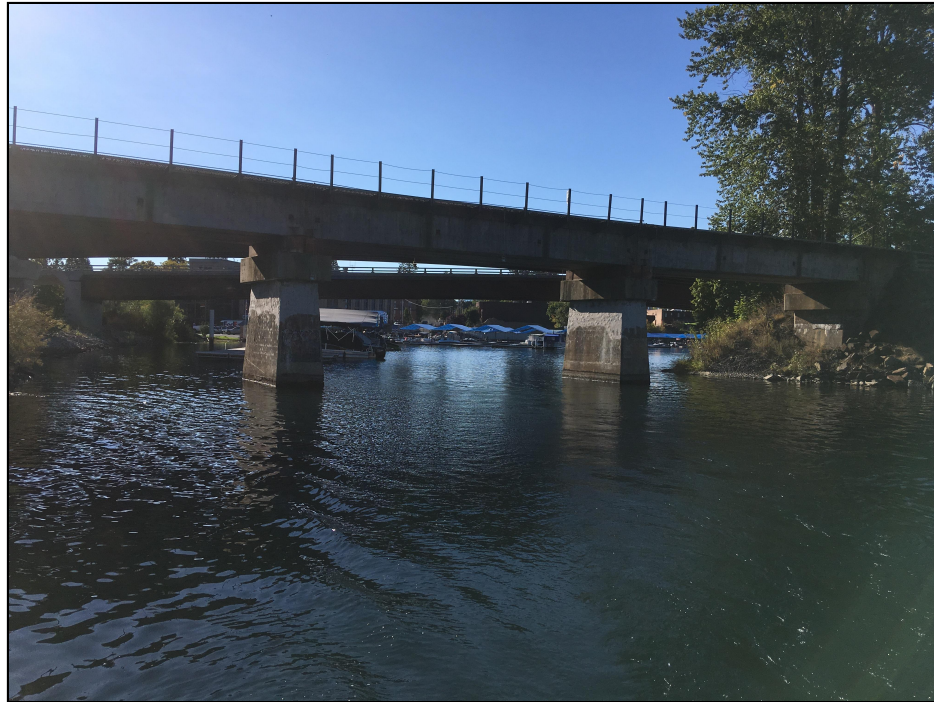
Bridge 3.1, East Elevation
